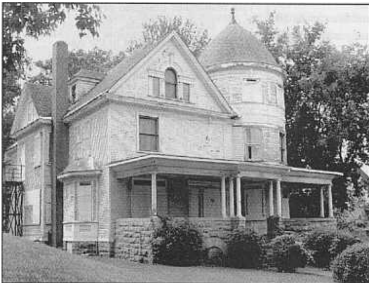
Local protected status has been granted to the former Jewish War Veterans' Post, but until renovation plans are implemented it is still endangered.
