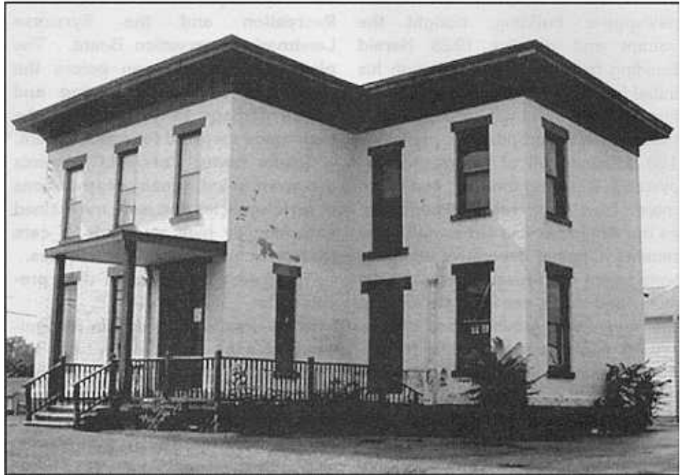
Harriet May Mills House on West Genesee Street is no longer in jeopardy of demolition following several well-orchestrated efforts in late June.
