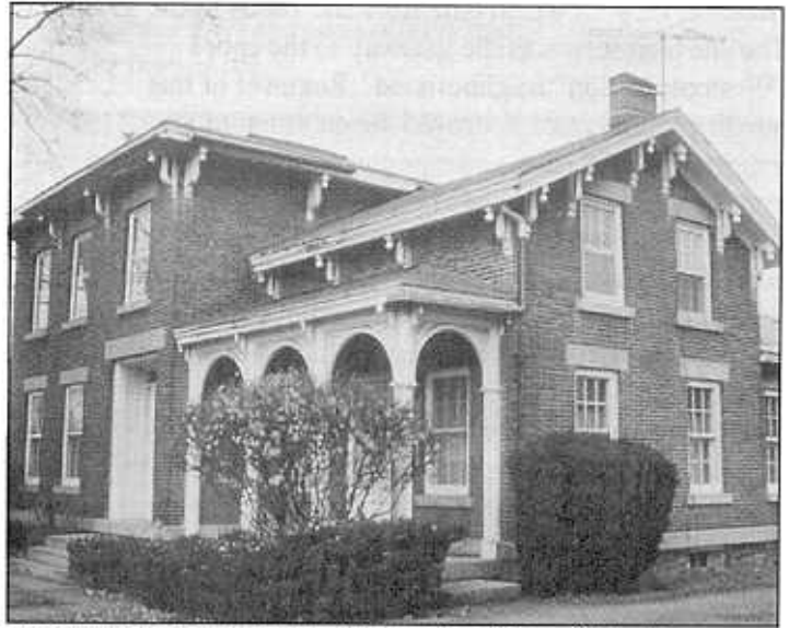
Ambrose Hine House, Nedrow, before demolition. Photo: Sam Gruber/PACNY
